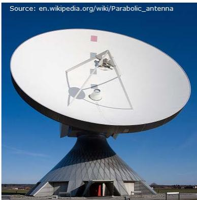
2. Radio telescopes are parabolic. In this case the dish is 32 metres across, with a depth of 7.2 metres.
